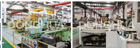
材料冷轧加工车间 Material cold rolling processing workshop
